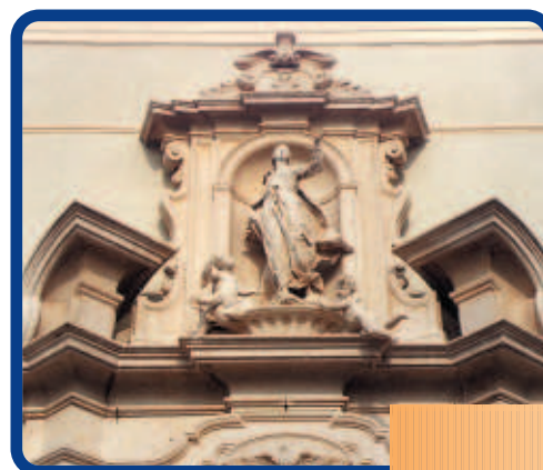
REMOVAL OF SMOG DEPOSITS AND GRAFFITI
